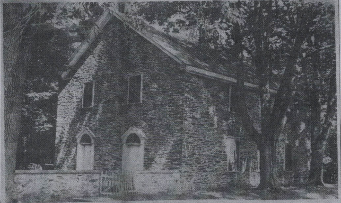
CIVIC, CHURCH and historic groups are united to try and save the old Locktown Baptist Church from being sold as a residence. Built in 1819, it is owned by the New Jersey Baptist Convention. A Flemington realtor holds an option on the property but says it's "not on market" now.
